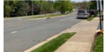
Existing sidewalk with grass buffer on east side, south of S. Four Mile Run Drive.
